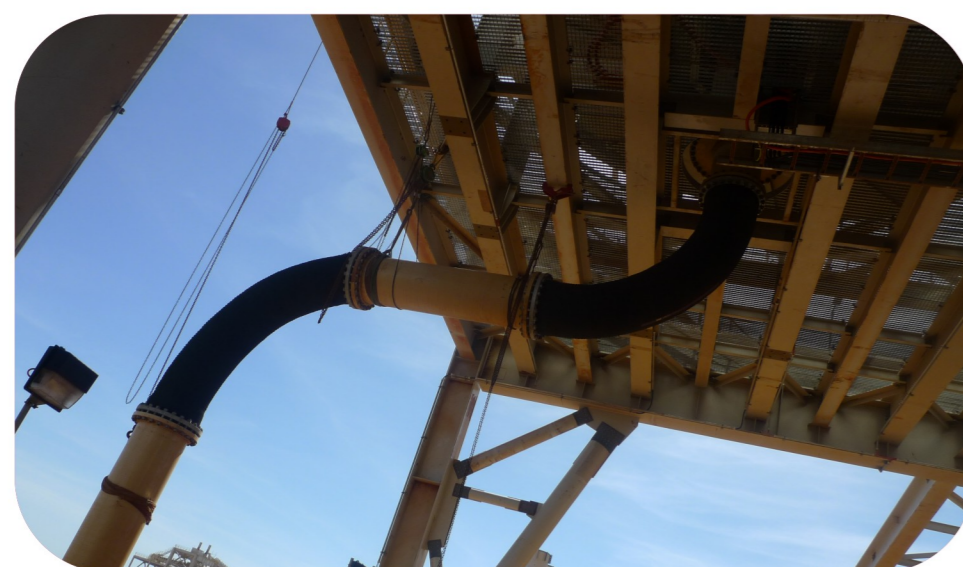
Rubber Mining Hose applied on site
